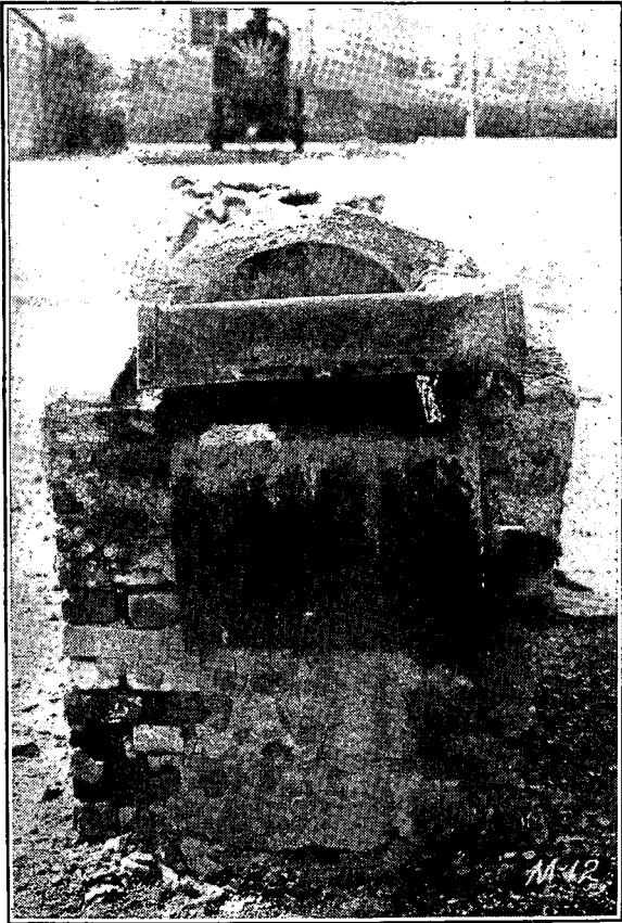
FIGURE 19.—Incline plane incinerator, end view.
