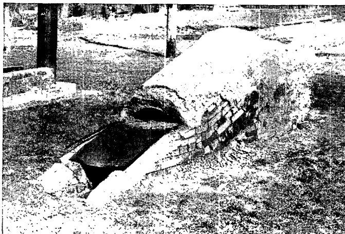
FIGURE 17.—Incline plane incinerator.
